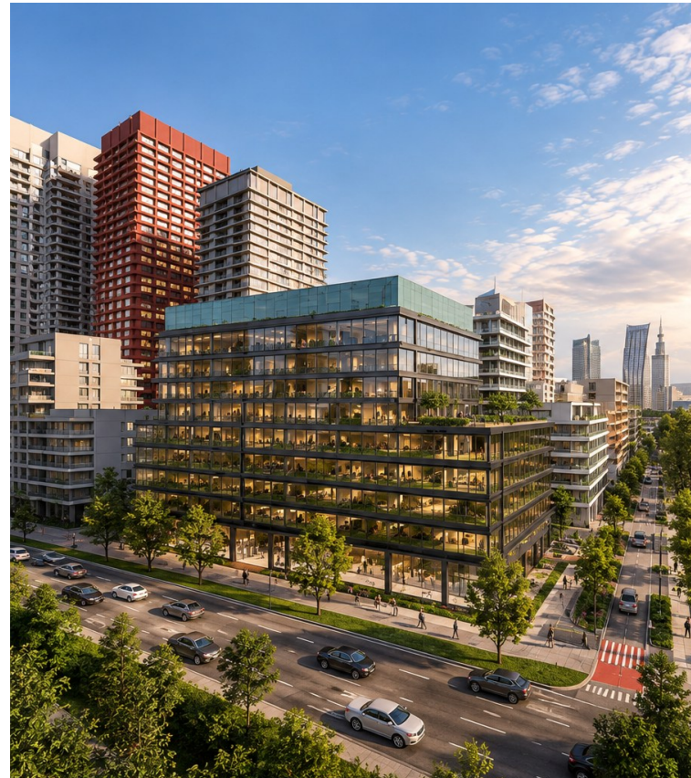
Towarowa 22 Warsaw next office phase
